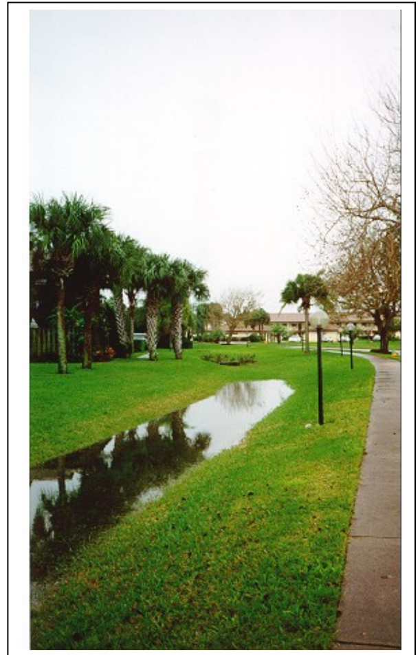
Stormwater swales help recharge groundwater and keep pollutants and debris out of our waterways.
